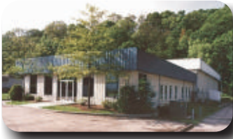
BENSHAW Inc. World Headquarters Glenshaw, PA
